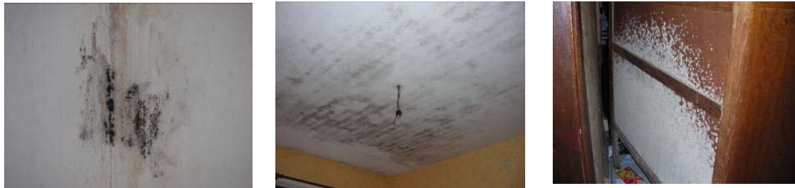
Figure 2 : Contaminated buildings (Source: Laboratoire de prévention des Pollutions Interieures (LPI), HVS, Mons, Belgium)
